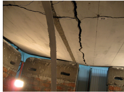
Fig. 8. Detail of the debonding failure taken after the end of the test on specimen RSC-01-FRP.
