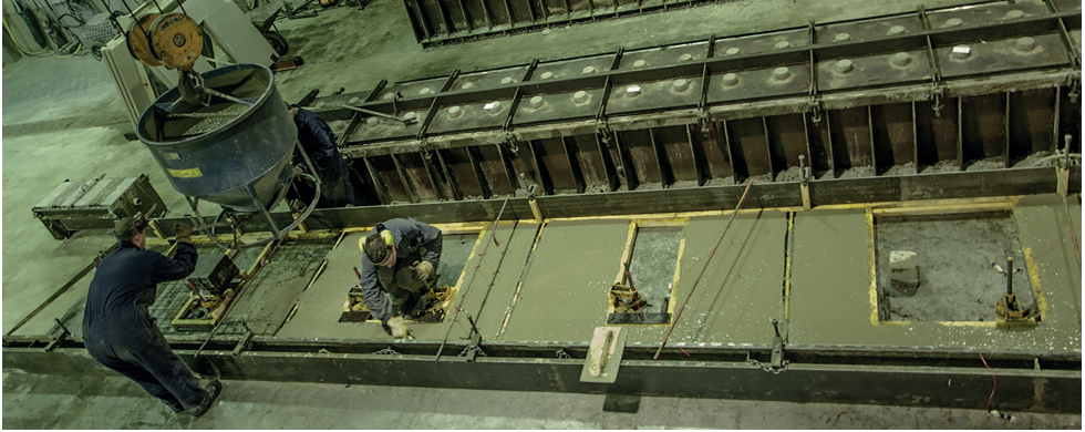
Figure 3.2 Long-line casting of walls
