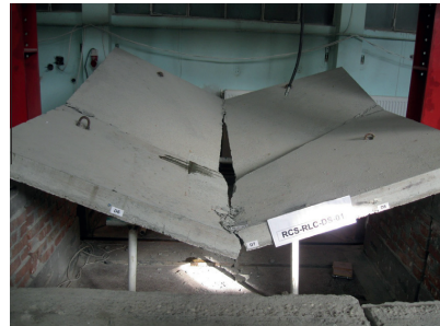
Fig. 9. Total collapse of the specimen RLC-01-FRP after testing.
